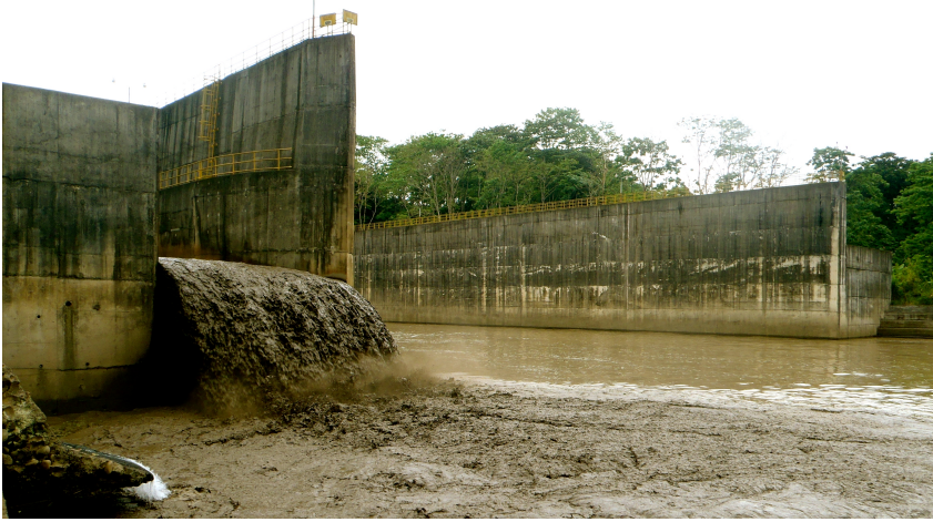
Figure 2.3: September flushing, downstream of Angostura spillway. Photo: S. Løvfall
