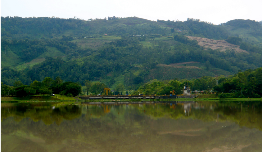
Figure 2.1: Gated spillway and intake structure, Angostura reservoir. Photo: S. Løvfall
